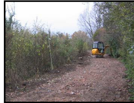
Construction of new Bridleway 25
